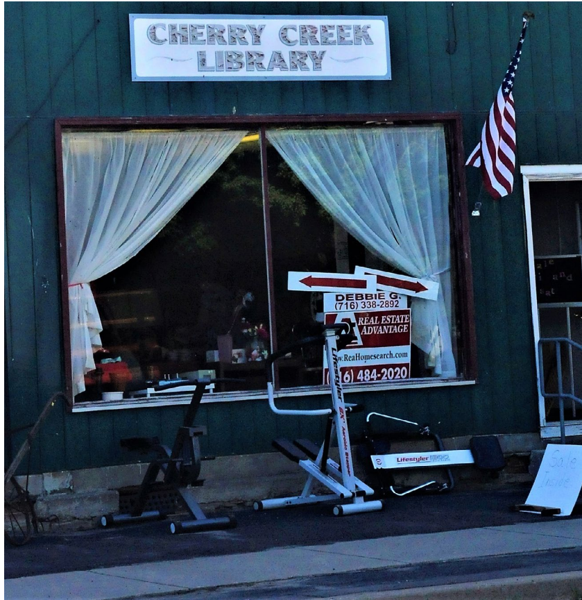
Properties along Main Street in Cherry Creek (Chautauqua County) show signs of aging and ill repair. Cherry Creek voted to dissolve in 2017.
